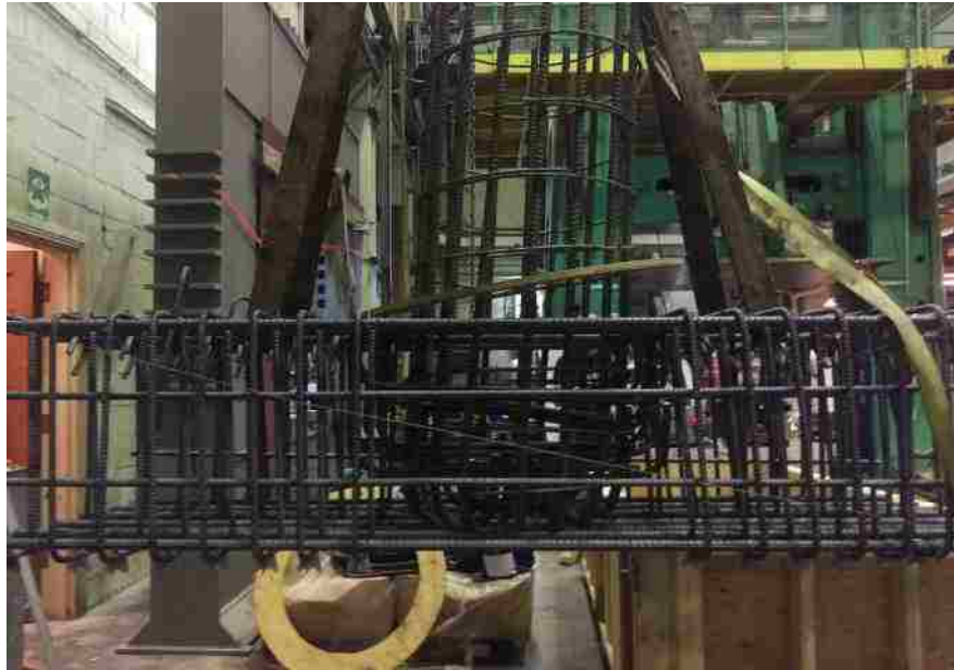
Figure 7-14. Reinforcement cage for cap beam being lifted into formwork for casting
