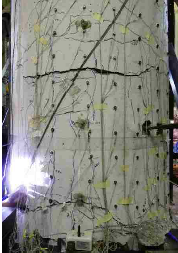
Figure 8-12. Very wide crack on north face, Series 8
