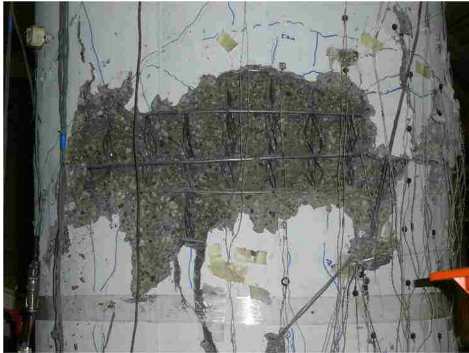
Figure 9-3. "Damaged Area" at end of testing showing concrete spalling, buckled strands and spiral deformation
