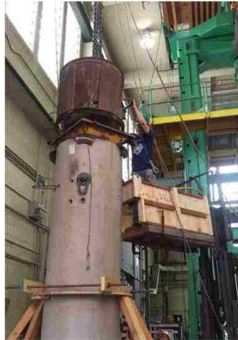
Figure 7-20. Casting plug inside of column
