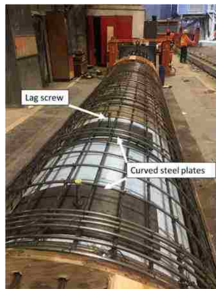
Figure 7-11. Hold-down plates used for sonotube during casting
